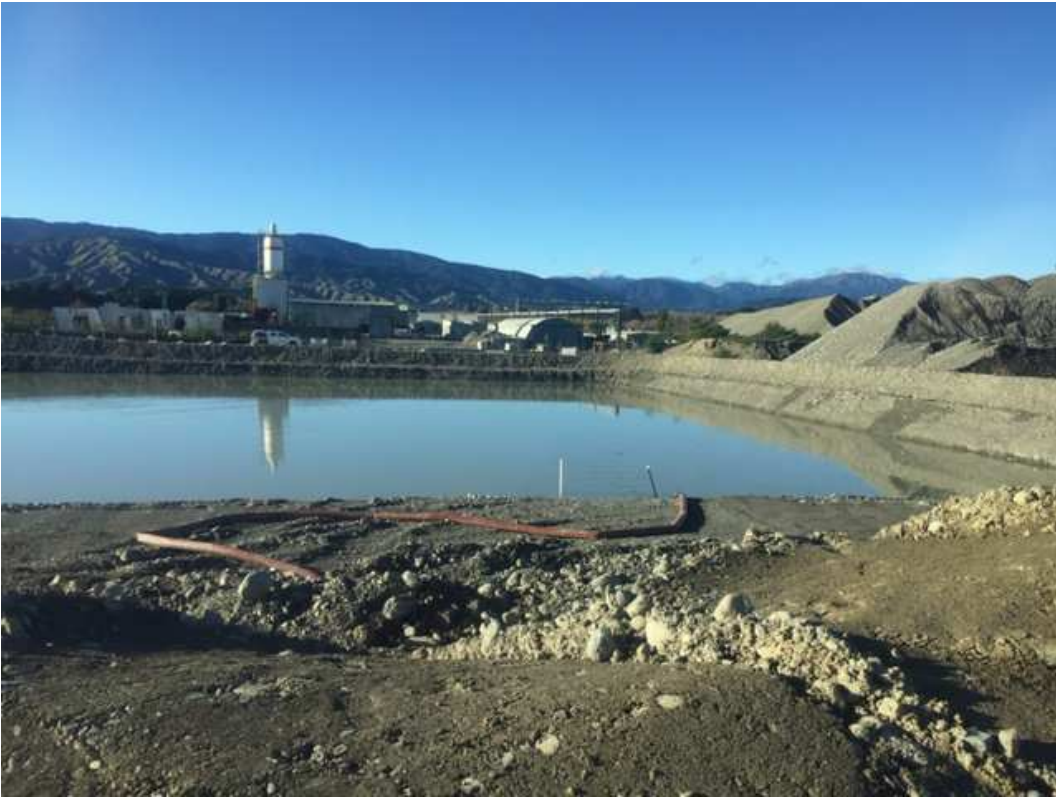
Figure 4: New secondary pond. Water does not discharge, but infiltrates to groundwater.
