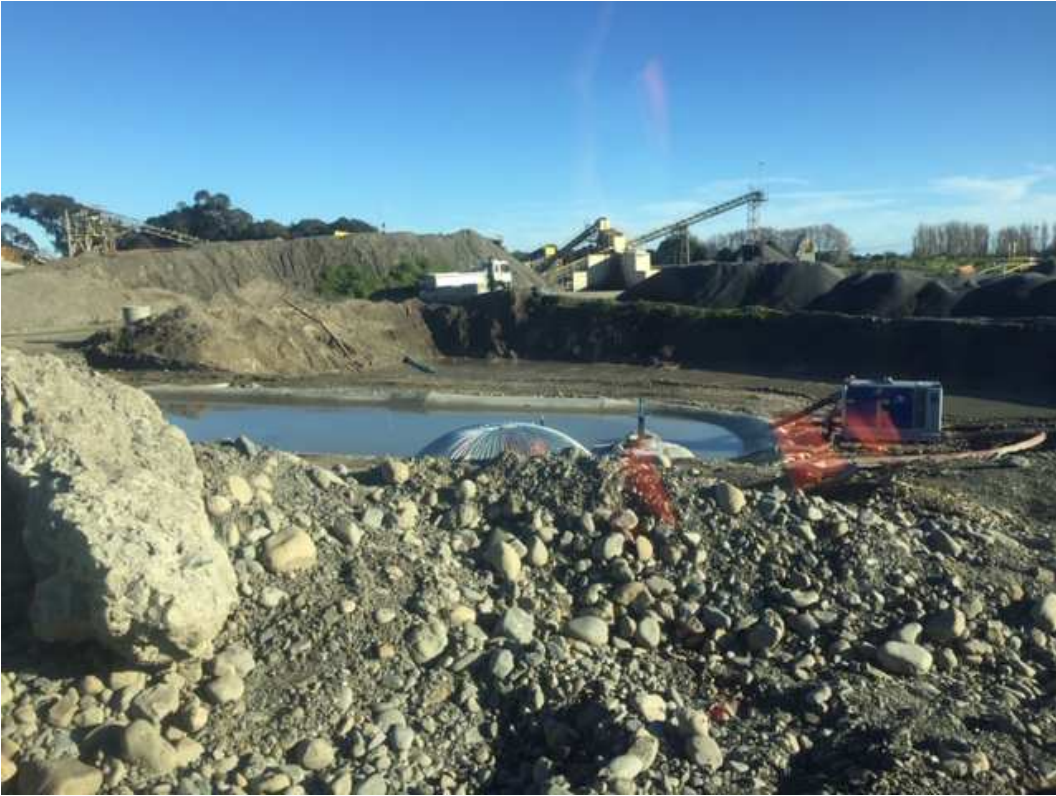
Figure 3: New concrete SRP (not required under consent WGN160103).
