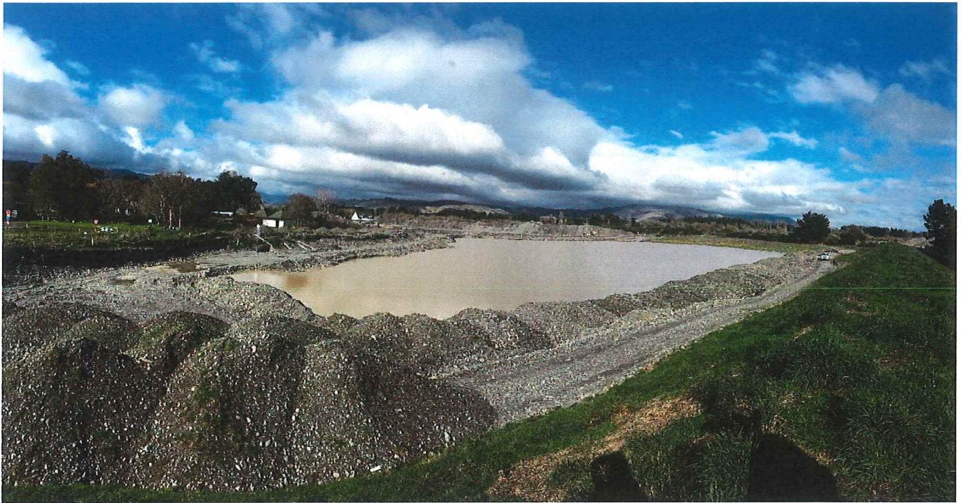
Stage 1A looking back to Stage 2 and large stockpiles in distance
