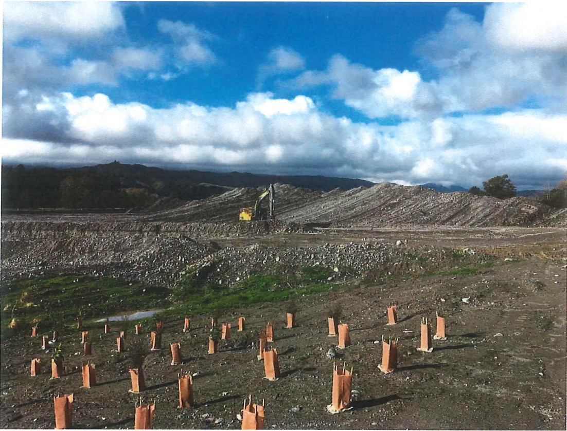
Rehabilitation plantings started in Stage 1A and Stage 2 stockpile in background
