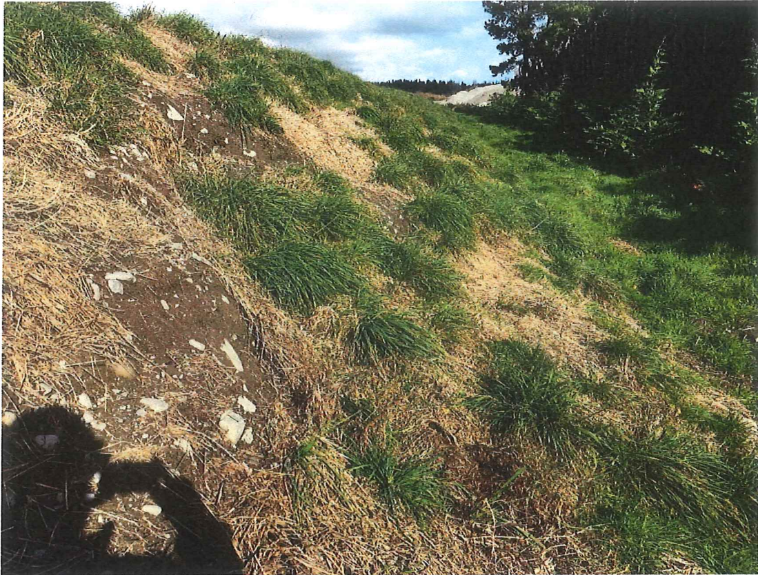
Slight movement in slump on Stage 1 bund noted.
