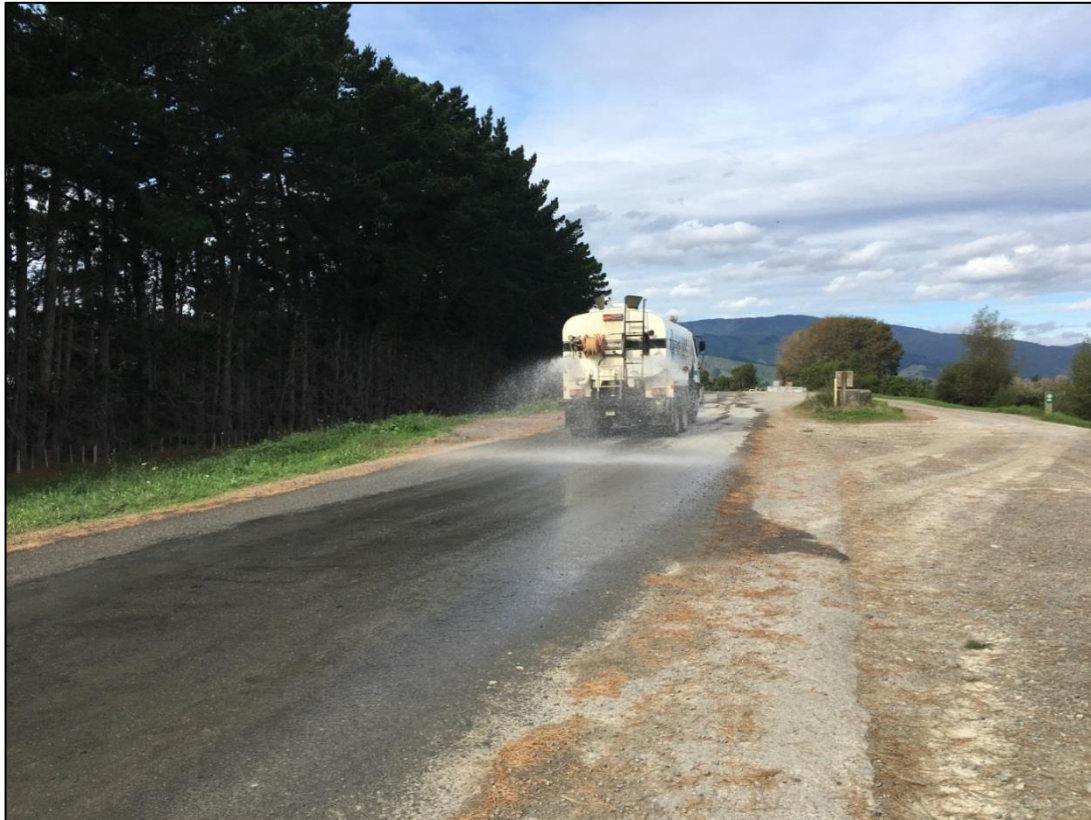
Figure 4 Water cart in operation
