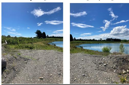
Stage two acoustic bund constructed and shaped ready for planting.
